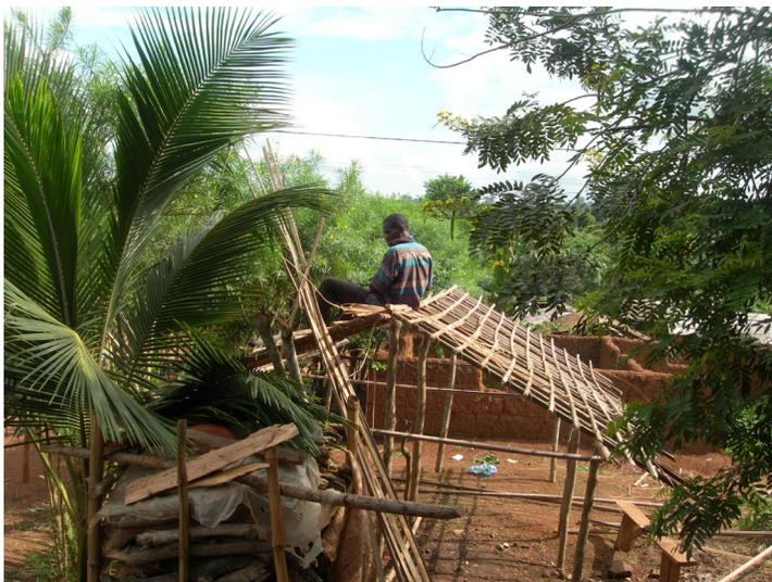
**HOUSE UNDER CONSTRUCTION IN DEPA, COTE D'IVOIRE.** First, the frame is constructed and all joints are tightened with fibers from a palm tree. Then the walls are packed with mud.
